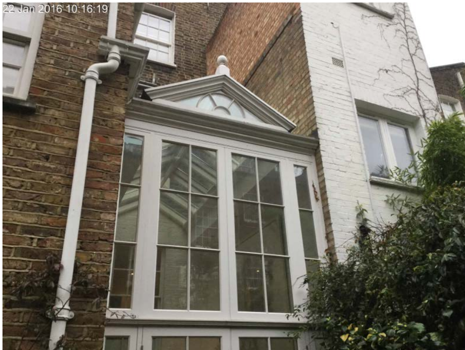
Rear elevation of 10 Northumberland Place
